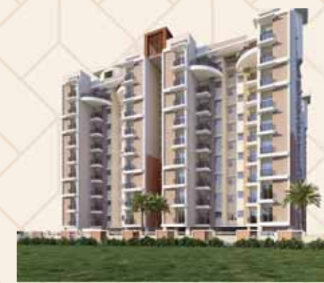
Protech Green Panjabari, Guwahati Aug'20 - Ongoing
